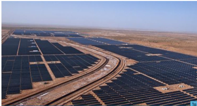
Fig: 3 Gujarat Solar Plant
